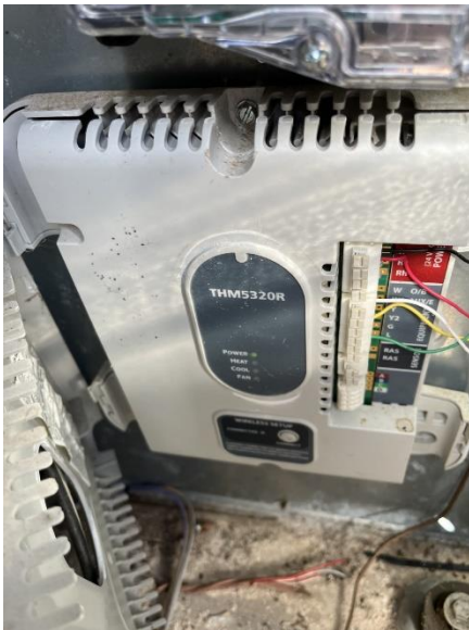
Replaced Power Supply Cord at Water Plant
